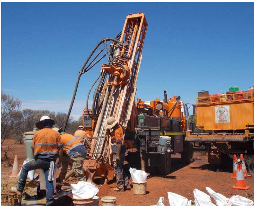
Plate 2: AC/RC Drill Rig at Indomitabile
